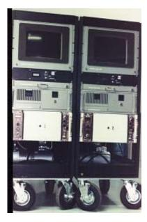
Cart-Mounted Control System for Stack Monitors
